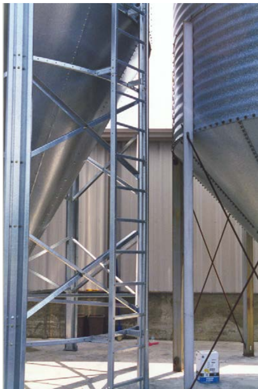
Figure 62 Side Ladder Assembled
